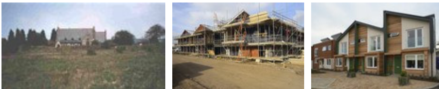
Photos 52, 53 & 54 - Former Linton Hospital. SixtyK Consortium: 2006
